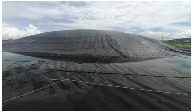
Fig7: The overview of earth pond and lagoon after covering HPDE for biogas production in Cambodia.
